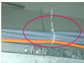
Excessively strong tightening fixing ties
